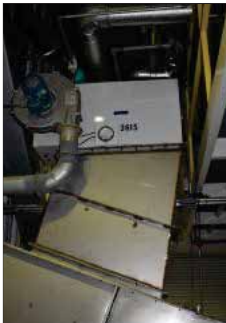
Above left: A special transition between pieces of equipment contains a spot filter for removing fines from the product flow. Above right: Hi-Vac vacuum systems powers cleanup throughout the plant. Below: Cleaver Brooks boiler is rated at 350 hp.
