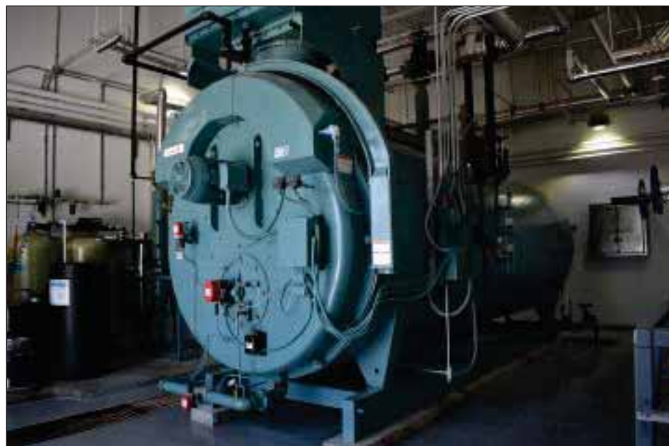
Above left: A special transition between pieces of equipment contains a spot filter for removing fines from the product flow. Above right: Hi-Vac vacuum systems powers cleanup throughout the plant. Below: Cleaver Brooks boiler is rated at 350 hp.
