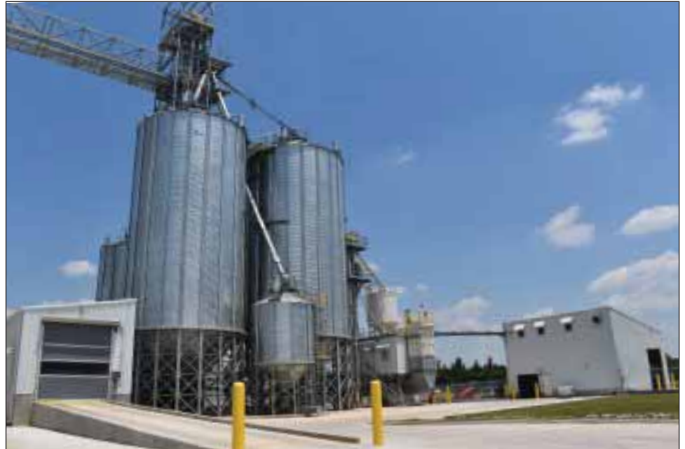
Small grain elevator holds locally-grown corn in two 40,000-bushel Chief hopper tanks with a Warrior 12-foot-x-18-foot-x-148-foot support tower and a 10-foot-x-8-foot-x-89-foot box bridge.
