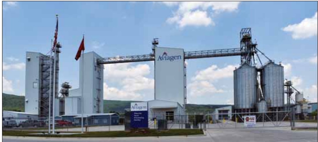
Aviagen, Inc.'s new 3,000-tpw poultry feed processing facility in Pikeville, TN features an enhanced level of biosecurity. Photos by Ed Zdrojewski unless otherwise indicated.
